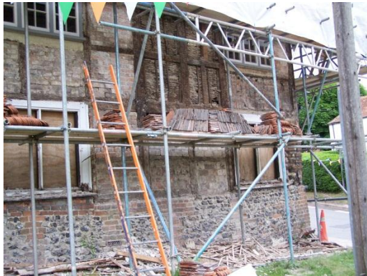
During renovation, showing exposed timbers
